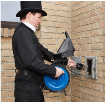
Fig. 25: Cable reel camera carried in front of the body
